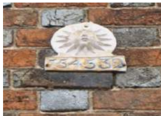
Picture 13. Another example elsewhere on the High Street of a metal Sun Insurance fire plaque. Can you find it? Such plaques were added to buildings to identify them as being insured by the company's fire brigade in the 18/19th centuries before the advent of municipal fire services.
