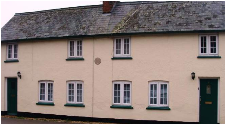
Picture 25. Nos. 1-3 Chapel End. Plaque reads These properties...were bequeathed by the Buntingford Almshouse Trust by Miss A Saggors of Buntingford . Note harmony achieved by windows of same design and doors painted same colour.
