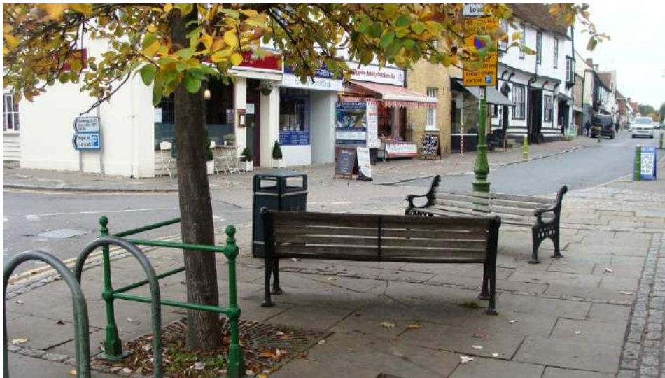
Picture 63. Minimum works involve repairs to one of the pair of seats.
