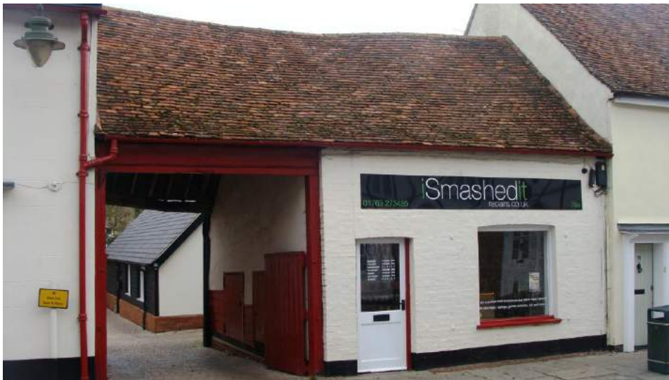
Picture 33. I smashed it repairs. Varied roofline adds to quality of the Conservation Area.
