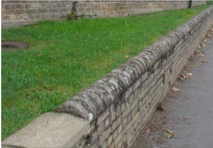
Picture 44. Curtilage listed low wall to Bridgefoot House. Modern concrete capping detail needs replacing.
