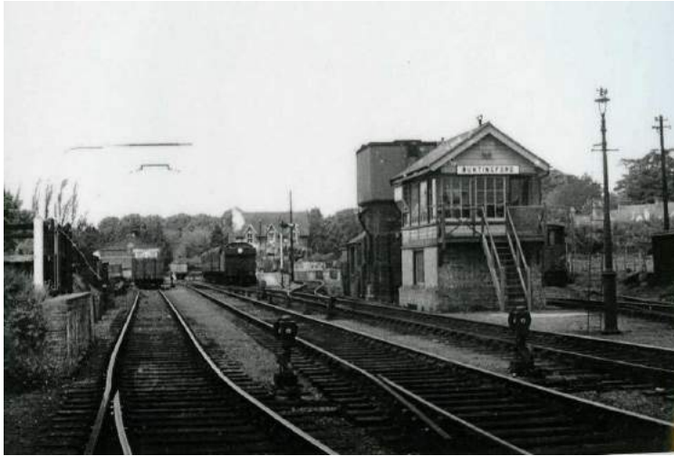
Picture 4. The railway station and branch line (1863-1965, freight). Now Fairfield Estate area. Reproduced from the collection of the late Philip W. Plumb and The Buntingford In Old Photographs Facebook page.
