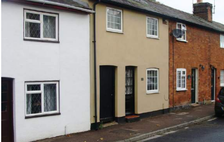
Picture 34. Nos. 1 - 7 Union Terrace. Despite alterations the mass of this terrace is visually pleasing and the buildings have interesting historical association.
