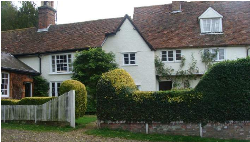
Picture 16. Layston Cottage, River Green - A large early 16th century Hall house with later additions.
