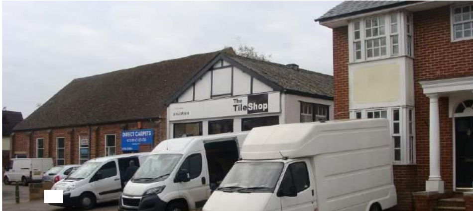
Picture 57. Site principally consisting of The Tile Shop and Direct Carpets is alien to the general alignment and historic qualities of the rest of the High Street. Its redevelopment to an appropriate use and at a sympathetic scale and alignment would be beneficial.
