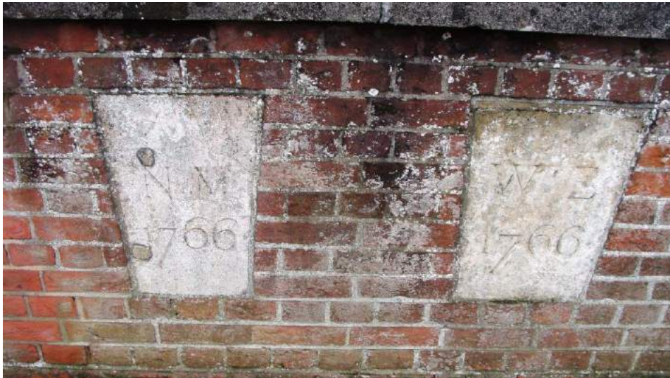
Picture 43. Historic plaques on bridge presumed to have formed part of an earlier bridge structure.
